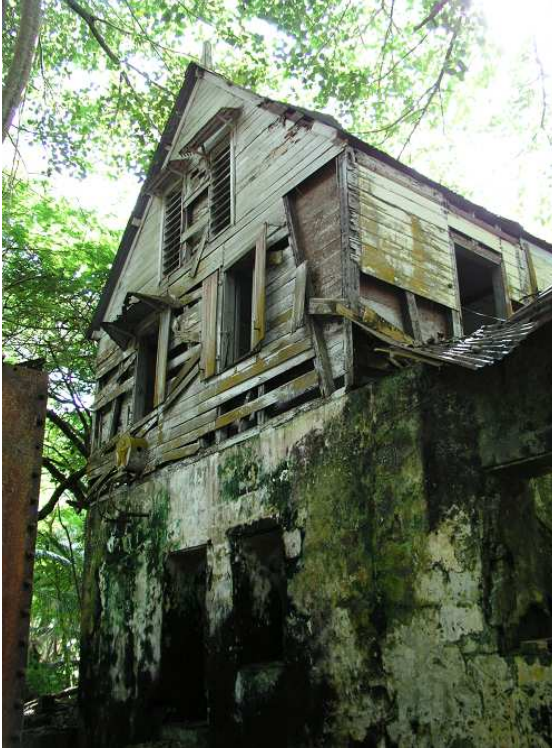
Figure 14. Left side of Peros Banhos Managers house on Ile de Coin in 2006. Remaining timber is rotten and floors are missing, as is some of the roof. Right: Ile de Coin jetty in 2006. The block where the photographer is standing is fairly solid but the shoreward 75% is rubble.
